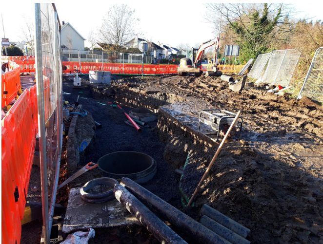
Above and below: N63 Majors Well Road Scheme - installation of underground services
